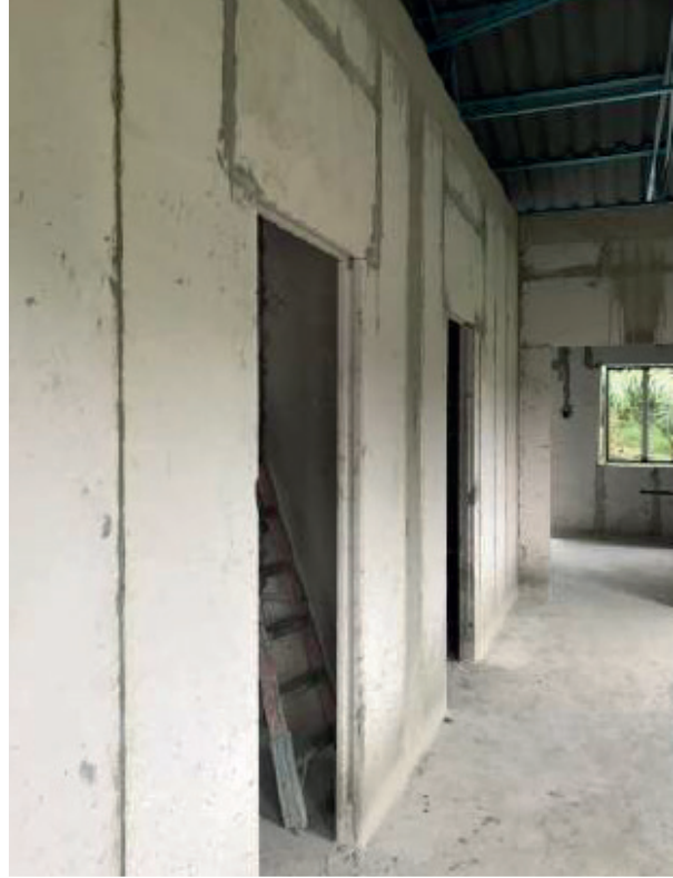
Installation IBS AAC Wall Panel for Private House at Banting Selangor.
