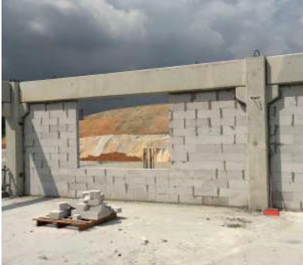
Installation IBS Lightweight Block for JKR Workshop, Wilayah Persekutuan.
