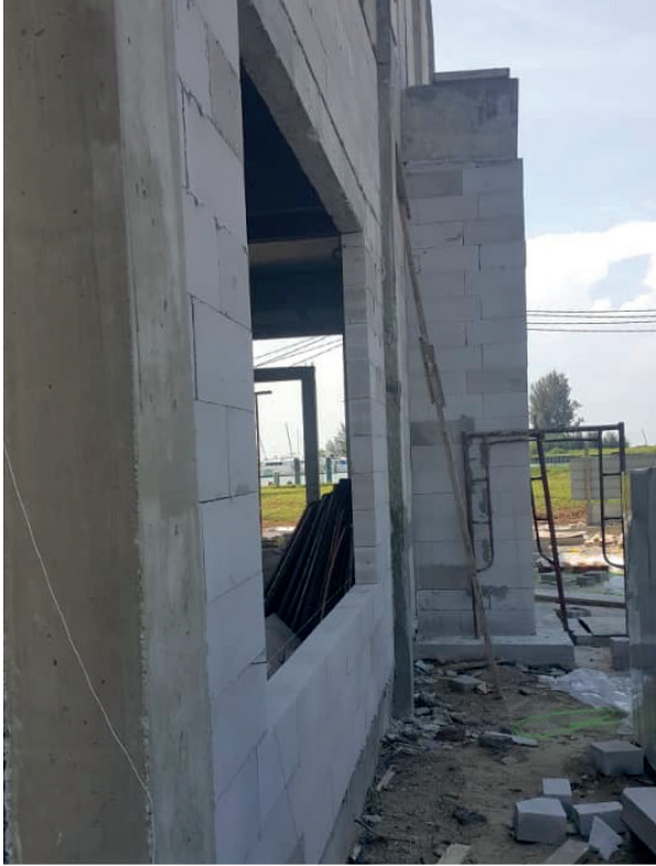
Supply and Installation IBS Lightweight Block for Two Units Private Bungalow Port Dickson, Negeri Sembilan.
