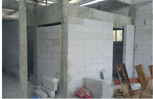
Supply and Installation IBS Lightweight Block for Two Units Private Bungalow Port Dickson, Negeri Sembilan.
