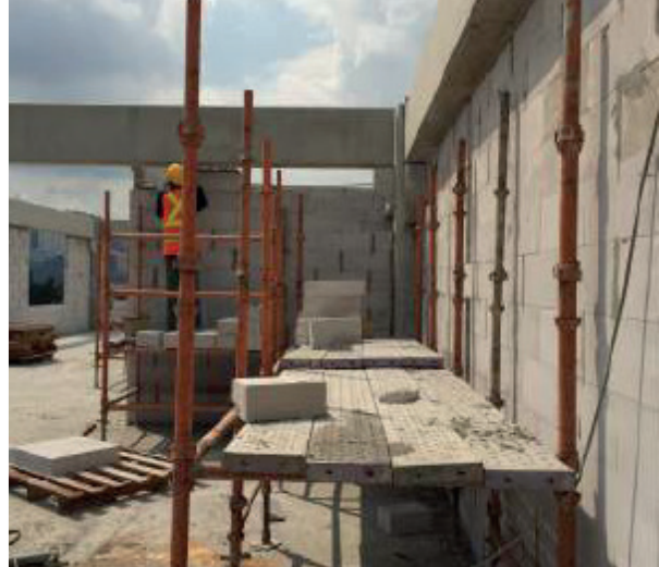
Installation IBS Lightweight Block for JKR Workshop, Wilayah Persekutuan.
