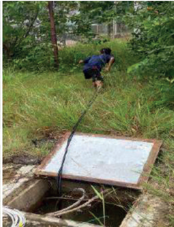
Installation Fiber Optical at Terminal Peluru 3, TUDM Labuan.
